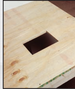
Cut the hole.
