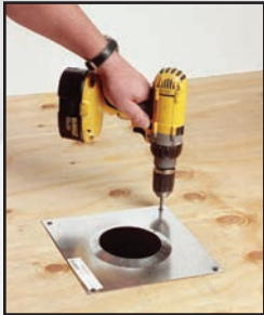
Mount SureGrip support plate.
