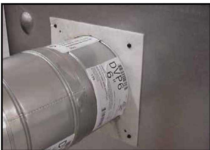
Figure 6.13 Attach the first vent section (it will snap into place). Slide the insulation gasket onto the vent section, up against the appliance and over the tabs. Use two self-tapping screws to secure gasket to outer wrap.
