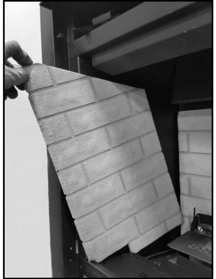
Figure 11.5. Install Left Side Refractory Panel
