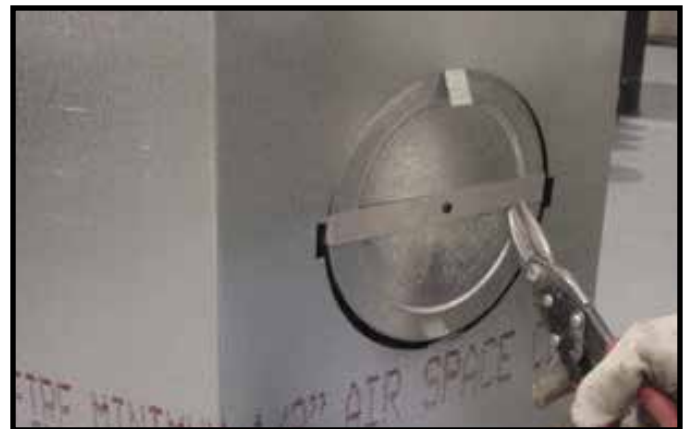
Figure 6.10 Cut the metal retaining band and fold the sides out.
