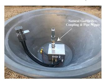
6. Install the Burner Pan. You will need to line up the Opening for the Pilot Burner with the Pilot Burner. You will notice that the hole in the center of the pan (for the pipe nipple coming from the Ignition Control Box) and the opening for the Pilot Burner are much larger than needed. This is done to make it easier to Install the Burner Pan. The large gaps around the pipe nipple and Pilot Burner will be covered with additional parts sent with the Burner Pan in Step 8 below.
